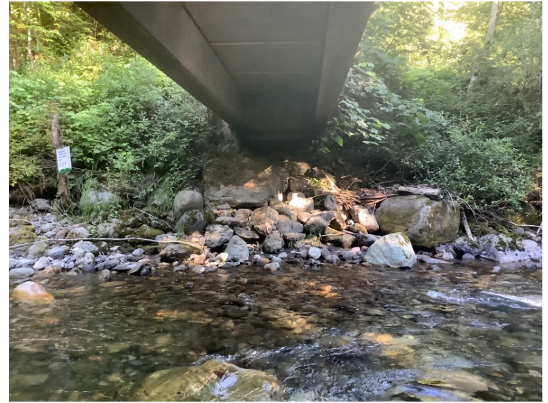
Left Bank Abutment when facing downstream
