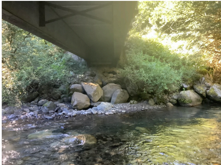
Right Bank Abutment when facing downstream
